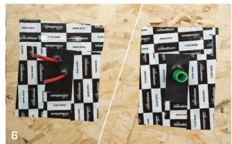
MANICA FLEX - TPU: SCELLEMENT D'UN TUYAU PASSANT
