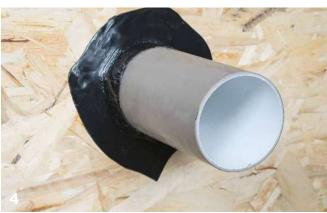
SCELLEMENT ASSEMBLAGE DANS LE NOEUD DE FIXATION AU SOL
