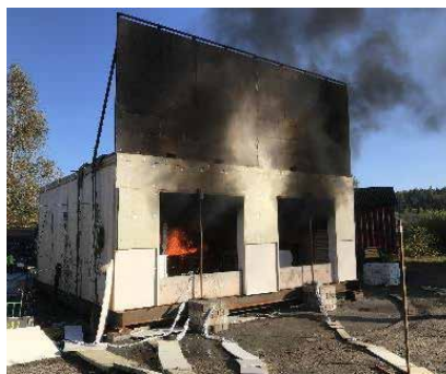
Photo of the compartment after switching on
