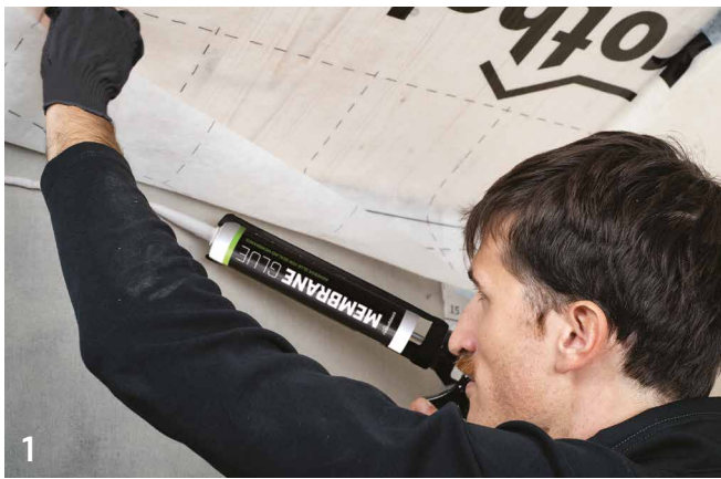
MEMBRANE CONNECTION TO ROOF - CONCRETE
