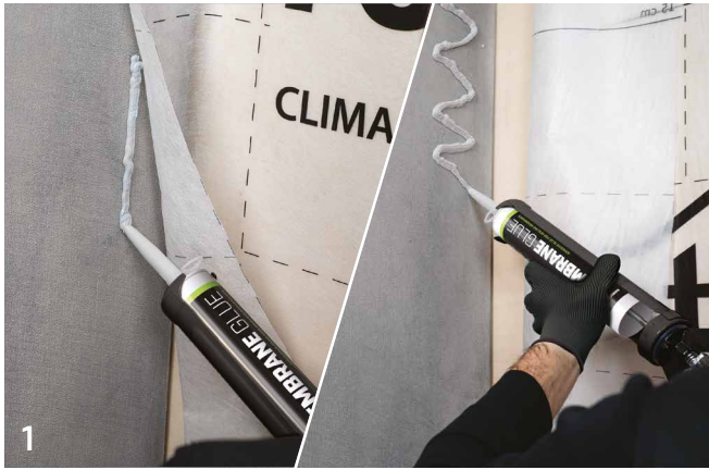
MEMBRANE CONNECTION TO WALL - CONCRETE
