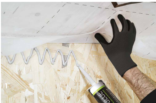
MEMBRANE CONNECTION TO ROOF - OSB
